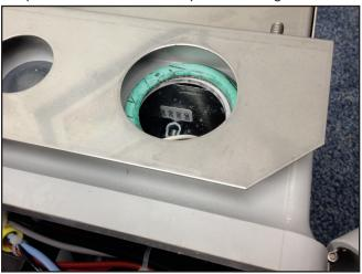
**5.** Screw conduit nipple (Item K) into conduit on Disconnect Housing Assembly (Item B) so that the Disconnect Housing Assembly extends toward the back of the heater. Do not fully tighten.
