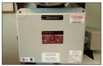
Remove Disconnect Switch Cover Assembly (Item A) from Disconnect Housing Assembly (Item B) by loosening four (4) capture screws.
