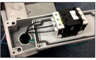
**14.** With disconnect installed, incoming power should be routed through disconnect enclosure conduit opening. Power wires should be installed in the remaining disconnect terminals and the ground wire should be spliced to the ground jumper wire using a wire nut.
