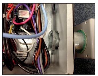
**4.** Place Neoprene gasket (Item M) over conduit nipple on outside of control panel housing.
