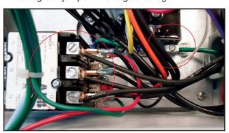
**13.** Install black jumper wires into disconnect terminals.
