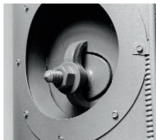
FIGURE 5 - INSPECT HAND HOLES FOR SCALE OR SLUDGE BUILDUP
